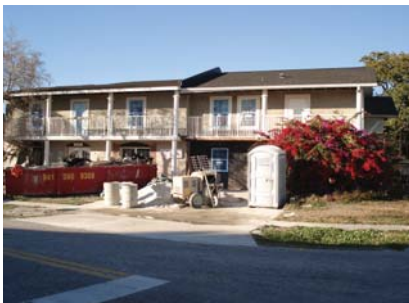
Restoration Roads Home Nearing Completion
